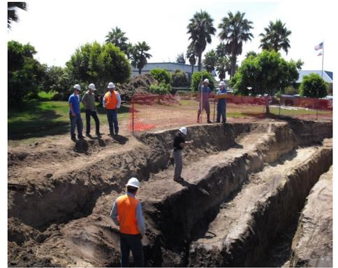
Trenching needed to satisfy requirements of a fault study for the wastewater treatment plant upgrade project. No fault lines were found clearing the way for construction on-site.
