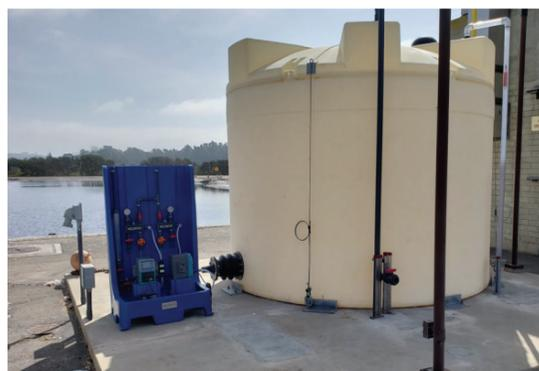
**Above Ground Diesel Storage Tank** - We operate 24 hours a day 7 days a week, even during emergencies. When there is no electricity we use diesel generators. We're replacing an aging diesel tank with a new and larger dual containment tank. The additional capacity will give the District the ability to operate for multiple days without utility power.
